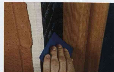
CONTEGA SOLIDO EXO windtightness tape may be used externally to seal windows or doors to block surfaces, for plastering later
