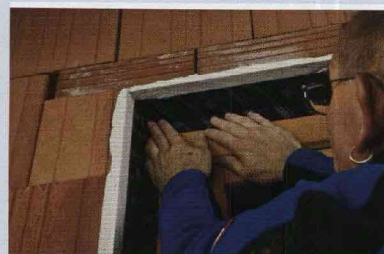
CONTEGA SOLIDO EXO windtightness tape may be used externally to seal windows or doors to block surfaces, for plastering later
