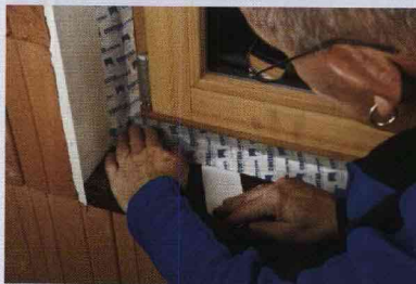
CONTEGA SOLIDO SL airtightness tape used internally to seal windows, doors or beams to block surfaces, for plastering later
