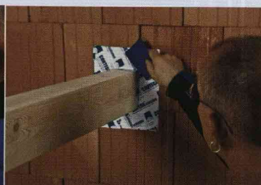
CONTEGA SOLIDO SL airtightness tape used internally to seal windows, doors or beams to block surfaces, for plastering later
