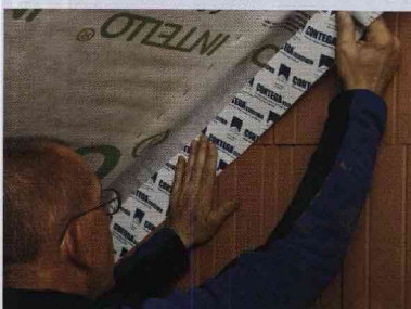
CONTEGA SOLIDO SL tape may also be used to seal vapour control layers (e.g. INTELLO PLUS) to block walls at wall plate level
