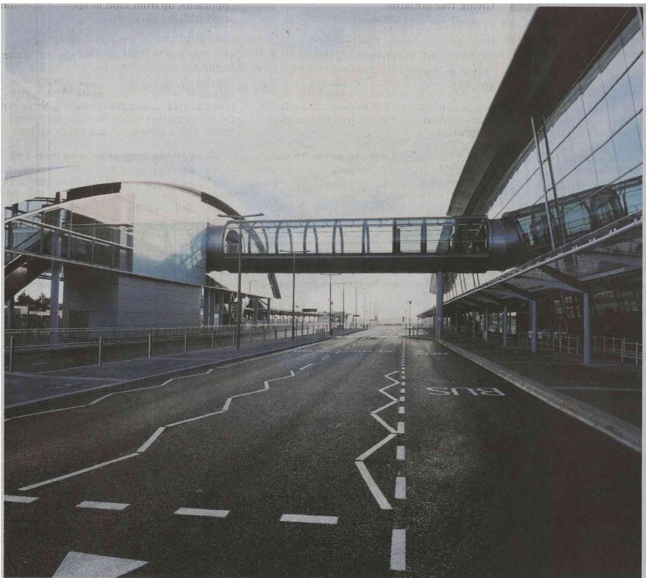
A key part of Ireland's infrastructure, Dublin airport's Terminal 2 was seen as by some as a 'white elephant' when it opened
