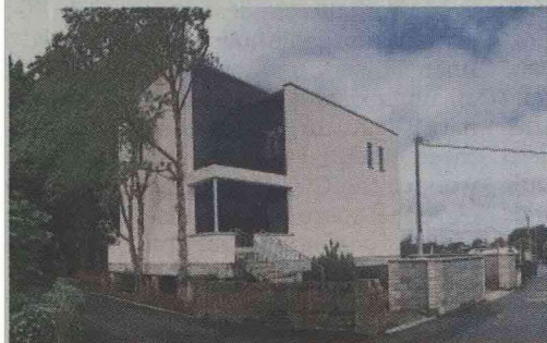
Donal Ryan's low energy house, Dublin Road, Thurles
