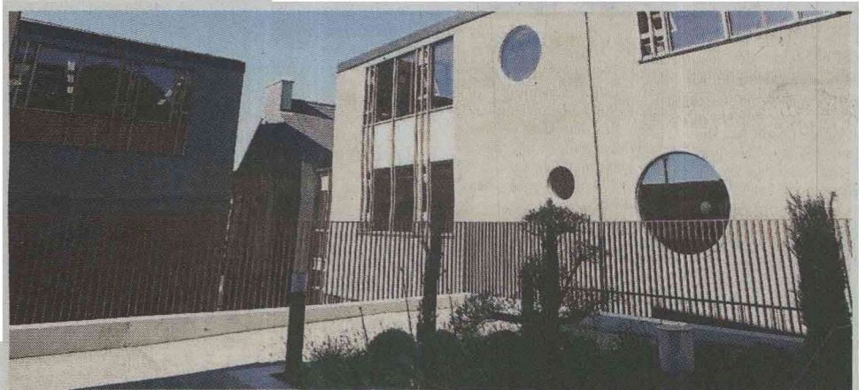
St Angela's College, St Patrick's Hill, Cork, was chosen in the Best Education Buildings category in this year's RIAI architecture awards.
